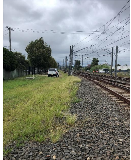
Image 4: View of Up direction Lookout at 47.622 KM Down cess.
