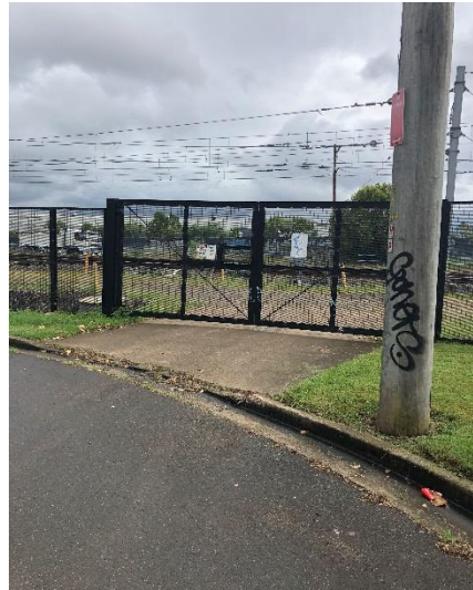
Image 3: Access/egress gate W00 47.649 D
