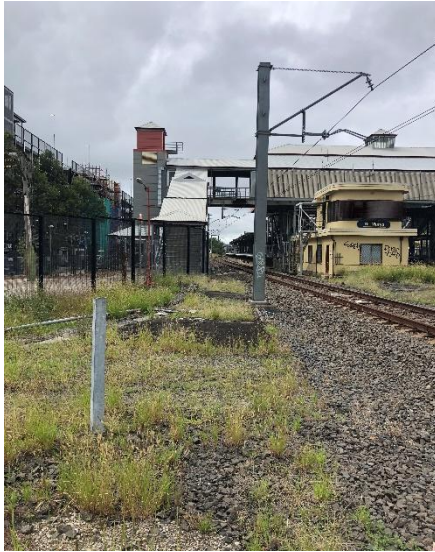
Image 3: View of Down direction Lookout at 47.570 KM Up cess.
