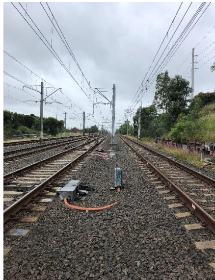
Image 3: View of Down direction Lookout at 46.948 KM 6 foot.
