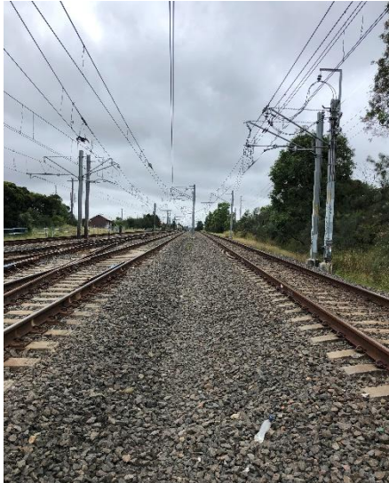
Image 1: View of Down direction Lookout at 46.913 KM 6 foot.
