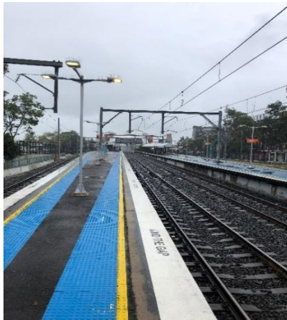
Image 1: View of Up direction Lookout City End of Platform 3 St Marys.
