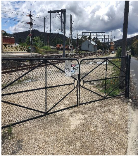
Image 3: Access/egress gate W00 155.328 D
