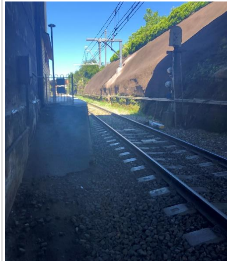
Image 4: Work Location at 96.6 Signal.
