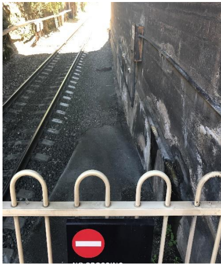
Image 3: Safe place for work at 96.6 Signal.
