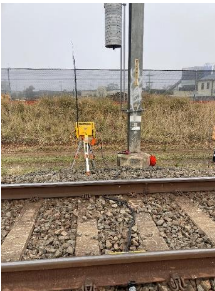
Image 1: Transmitter and sensor installation location
