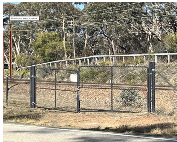
Image 2: Sensor access using access gate W00 116.782 U
