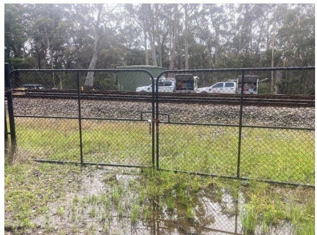
Image 2: Sensor access using access gate W00 114.511 D
