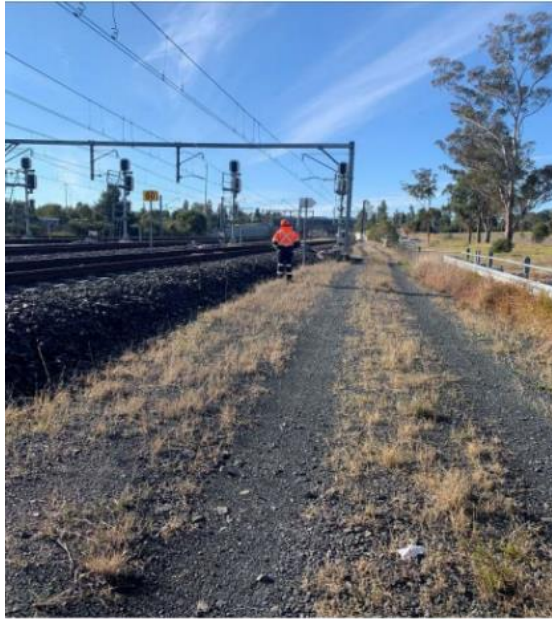
Image 3: Lookout in Down cess near LE 31 signal looking for approaching down rail traffic
