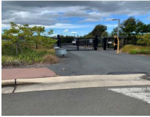
Image 7: Access to Leppington Stabling Yard off McCann Rd
