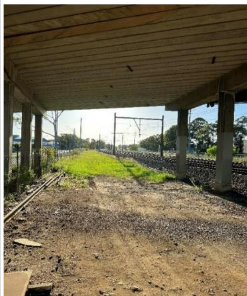
Image 4: View towards Leightonfield Station
