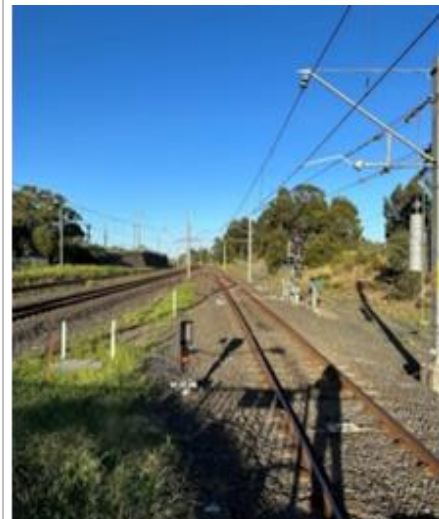
Image 4: View of worksite towards Carramar station
