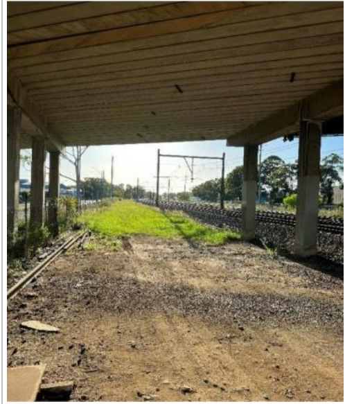
Image 4: View towards Leightonfield Station
