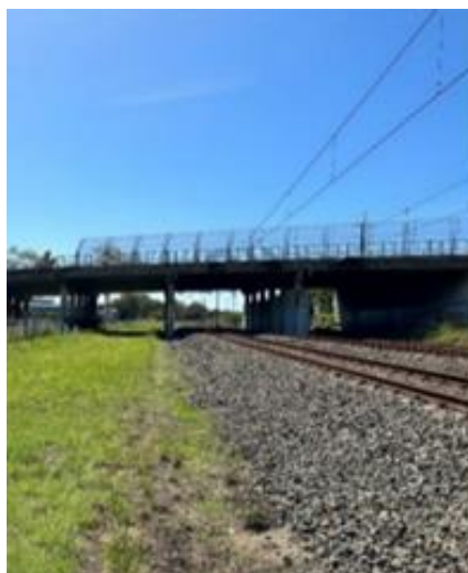
Image 3: View of worksite towards Leightonfield station
