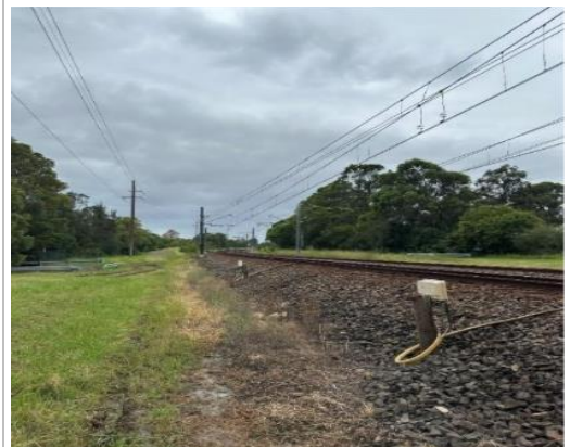
Image 4: View of worksite towards Panania station Facing the Up direction
