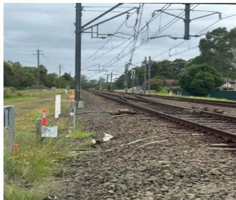
Image 3: View of worksite towards Panania station facing the Up direction
