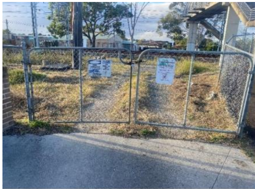
Image 1: Access gate M25 23.827U adjacent 15 Forest Rd, Up side at the city end of East Hills Station
