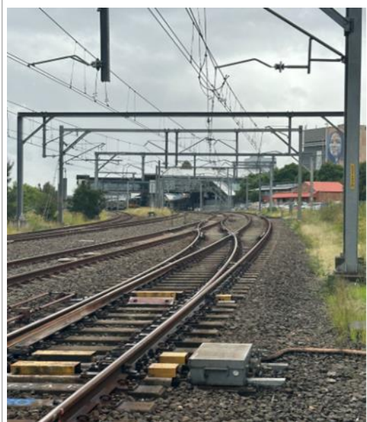
Image 4: view of worksite towards Liverpool.
