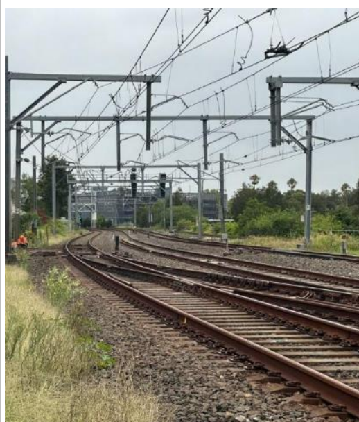
Image 3: View of worksite towards Warwick Farm
