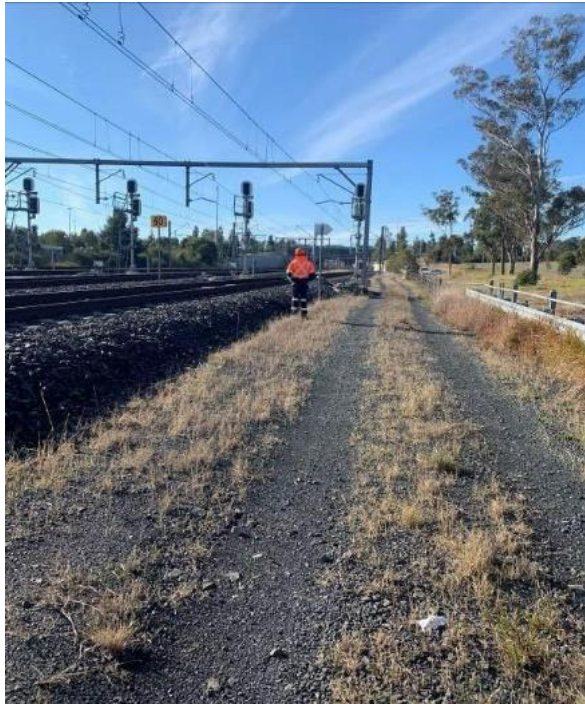
Image 3: Down cess near LE 31 signal towards Leppington Station.
