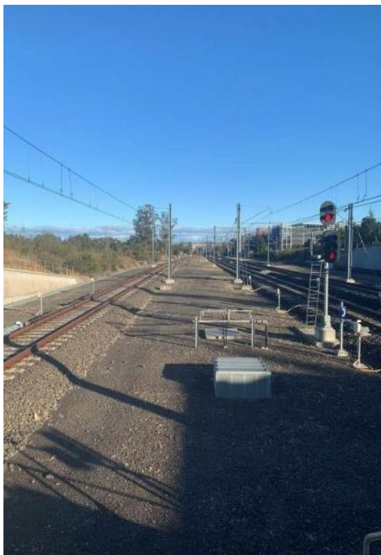
Image 5: View from countryside of Leppington station towards Leppington yard
