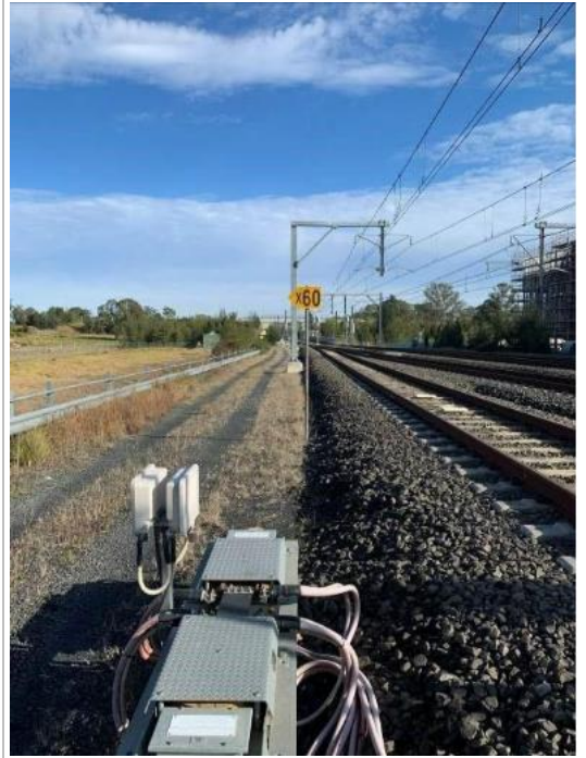
Image 4: Down cess near LE 31 signal towards Leppington Yard.
