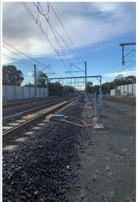
Image 6: View from Leppington yard towards Leppington station
