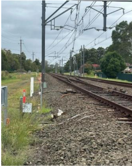
Image 3: View of worksite towards Panania station facing the Up direction.
