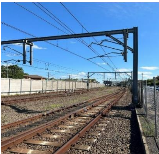
Image 3: View of worksite towards Cabramatta station
