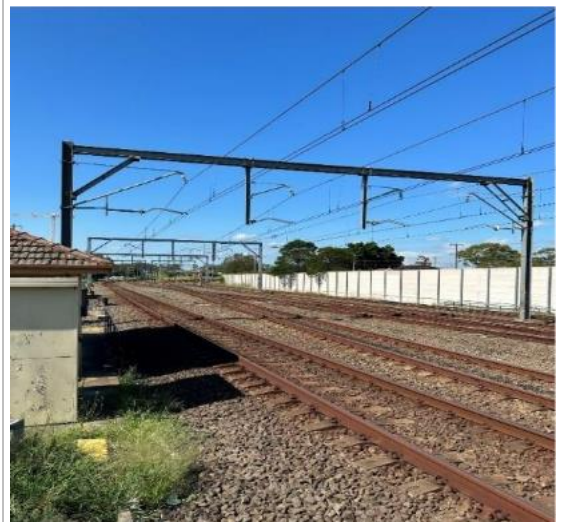
Image 4: View of worksite towards Canley Vale and Carramar stations
