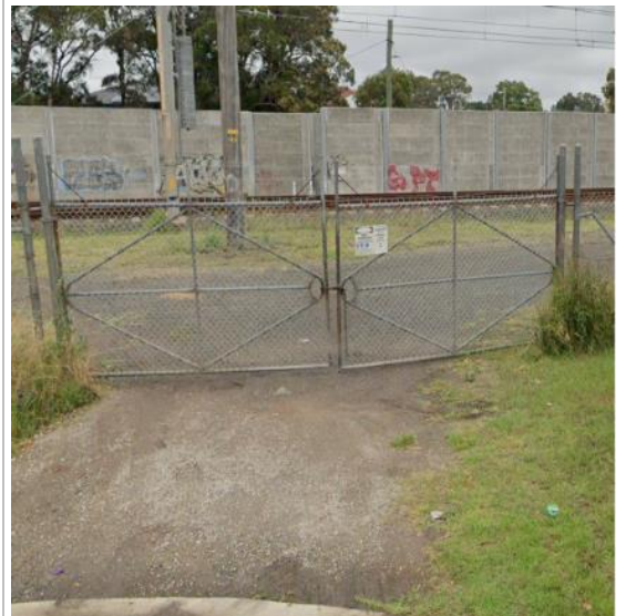
Image 2: access gate S00 27.519 U West street
