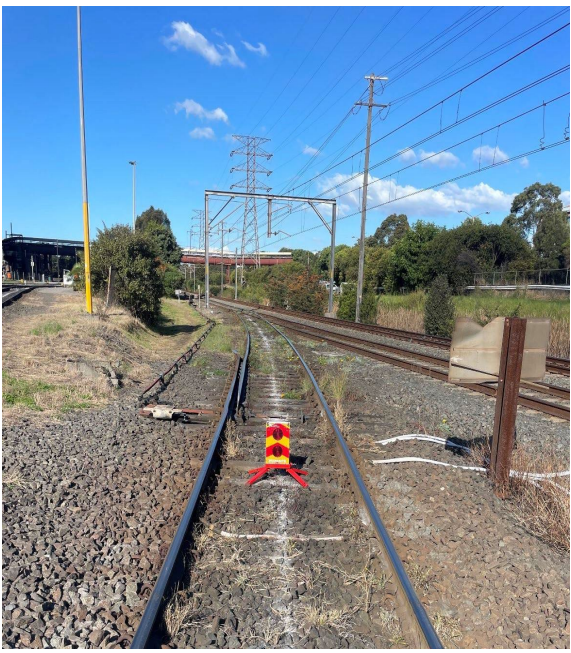
Image 4 Worksite Protection Marker placed clear of 531 Points (531 points clipped and locked by BlueScope Road Control).
