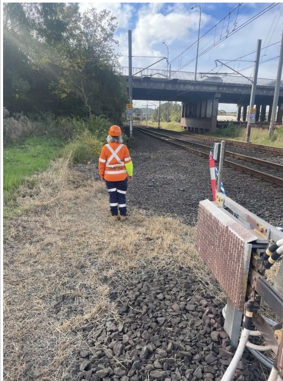
Image 1: Wollongong Side of worksite facing Wollongong
