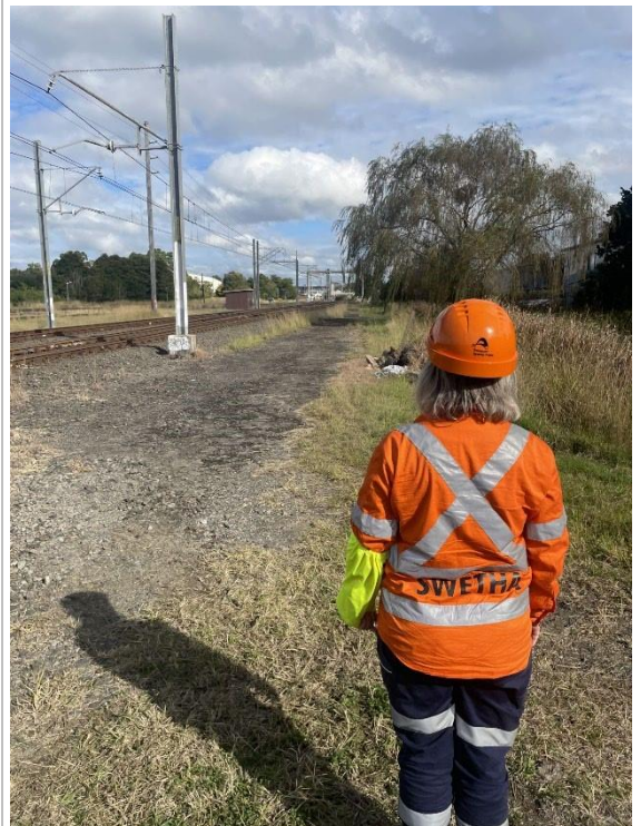
Image 2: Wollongong end of the worksite facing Dapto
