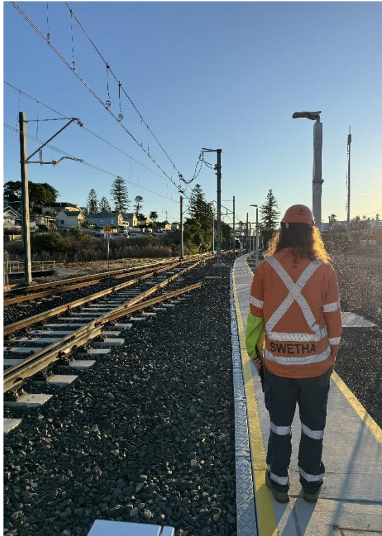
Image 3: Lookouts view from Down Cess adjacent to 54 points facing Wollongong
