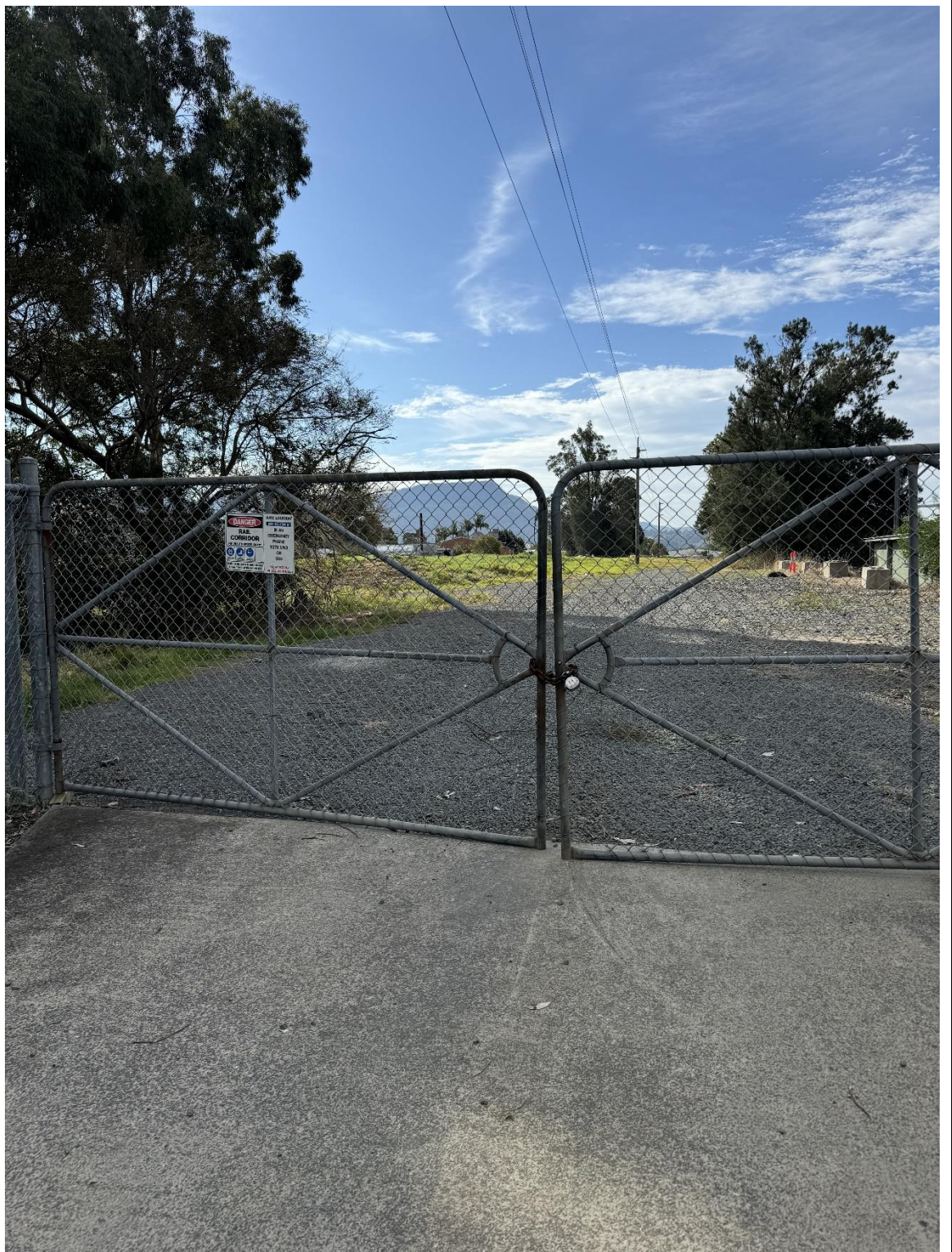
Image 8: Access Gate 100 95.134 U on the Up side off Bong Bong RD Dapto
