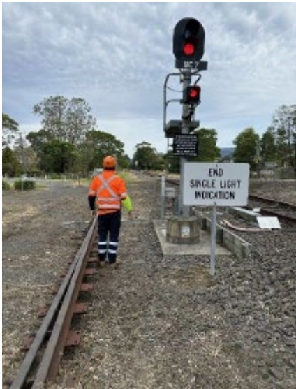
Image 5: View of Up direction Lookout at 141.197 KM
