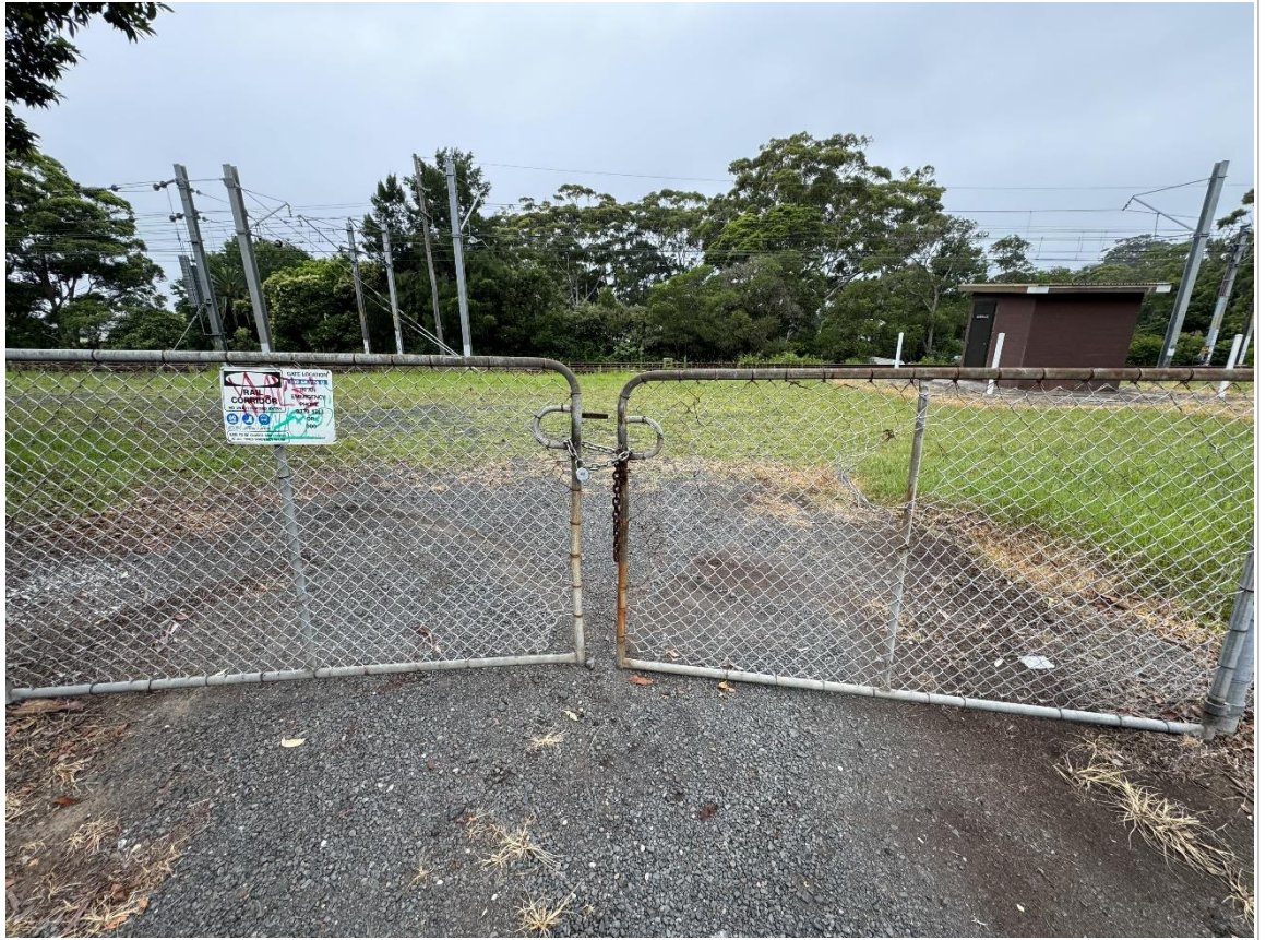
Image 3: Access Gate 100 68.376 at Austinmer on the Up side. Double gate on Railway Ave Austinmer
