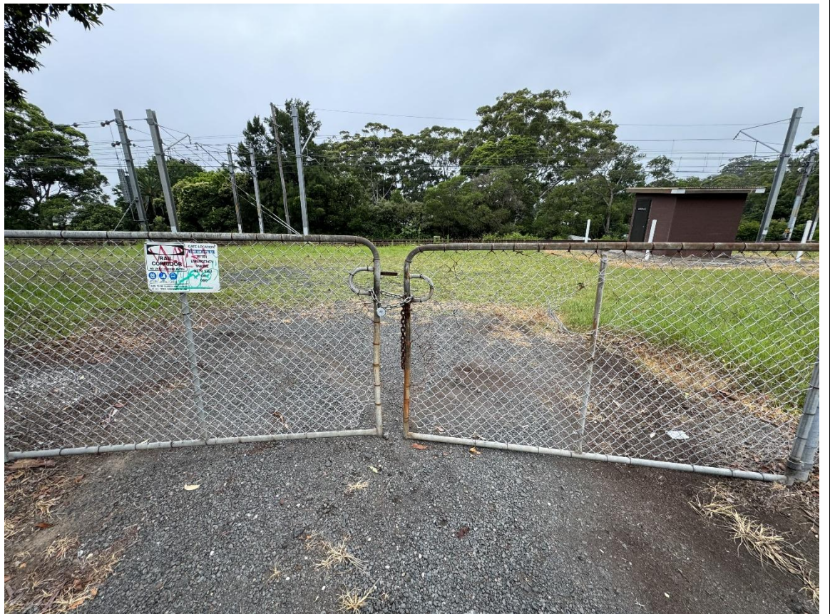
Image 5: Access Gate 100 68.376 at Austinmer on the Up side. Double Gate in the middle Railway Ave Austinmer
