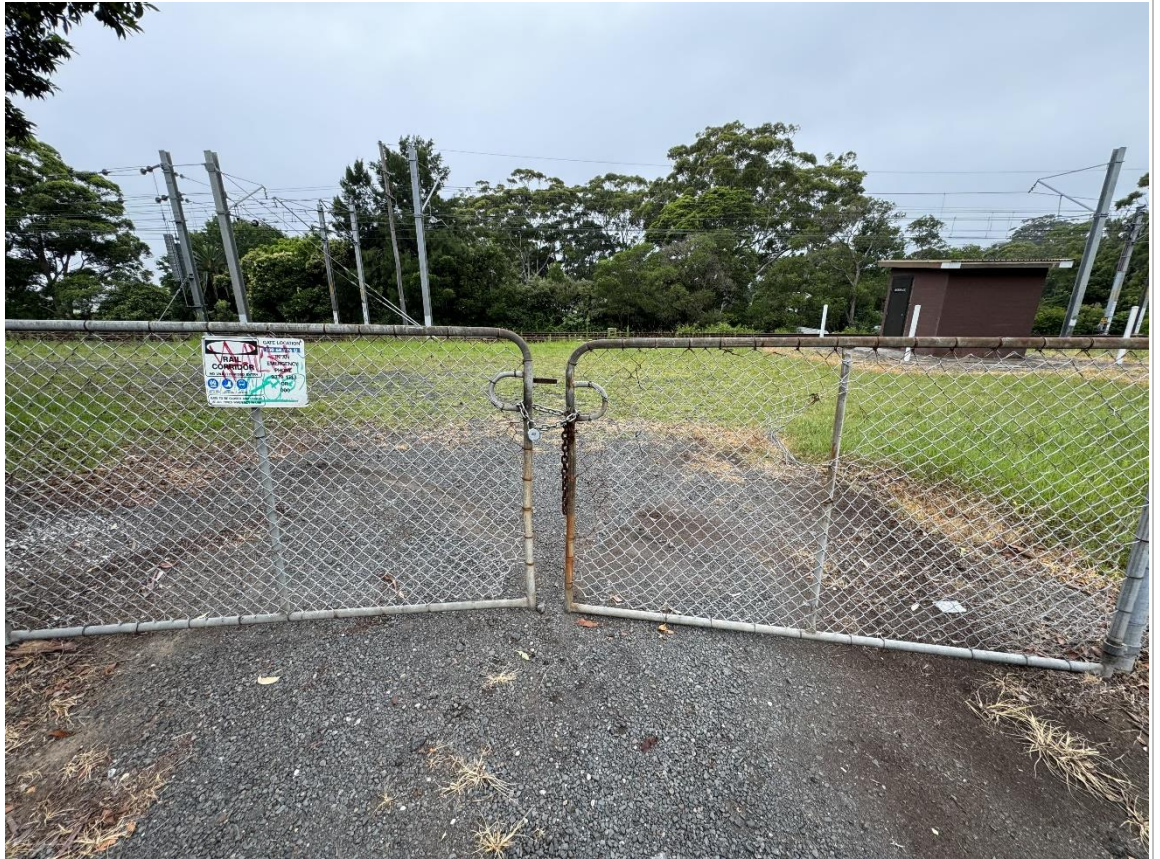
Image 5: Access Gate 100 68.376 at Austinmer on the Up side.
