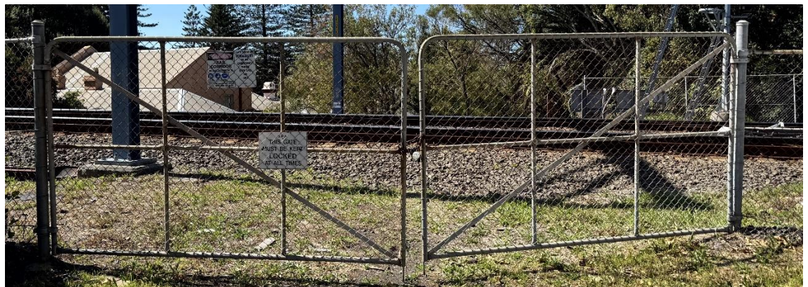
Image 2: Access gate 100 119.070 U on Railway Parade.
