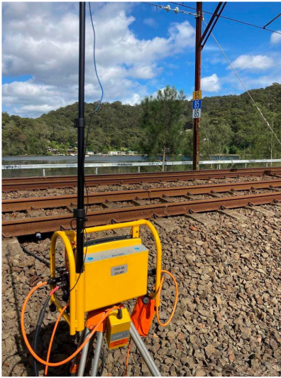
Image 1: Sensor and transmitter installation location
