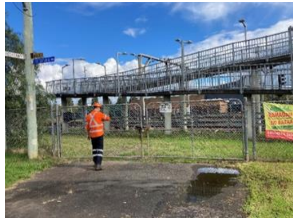
Image 2: Sensor access using access gate N00 49.763 D
