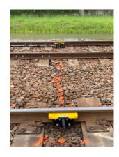
Image 1: Sensor and transmitter installation location
