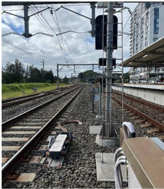
Image 3: View towards 1-4 Platforms Tempe
