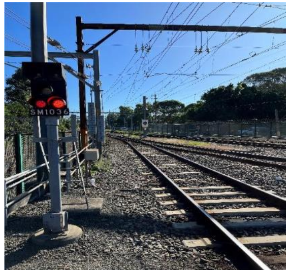
Image 6: View towards 1 & 2 platforms Mortdale. SM1036 signal indicating the start of the Signaller's limits.
