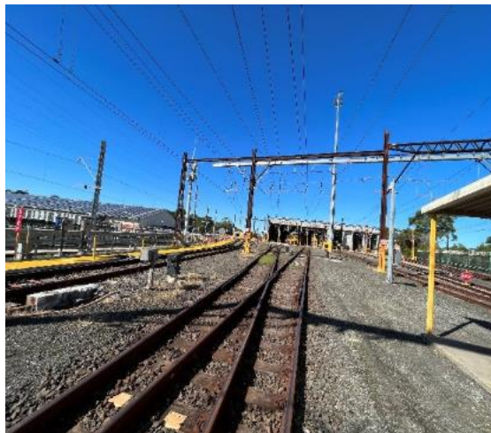
Image 7: View towards MMC Shed. Inclusive of STOP signs indicating the end of the signaller's authority and the beginning of the Yard Master's authority.
