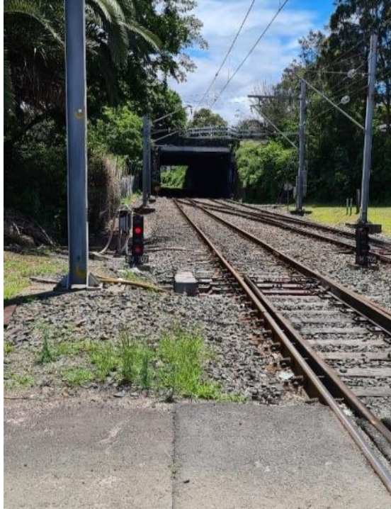
Image 1: View towards Up & Down Goods between level crossing & Bridge
