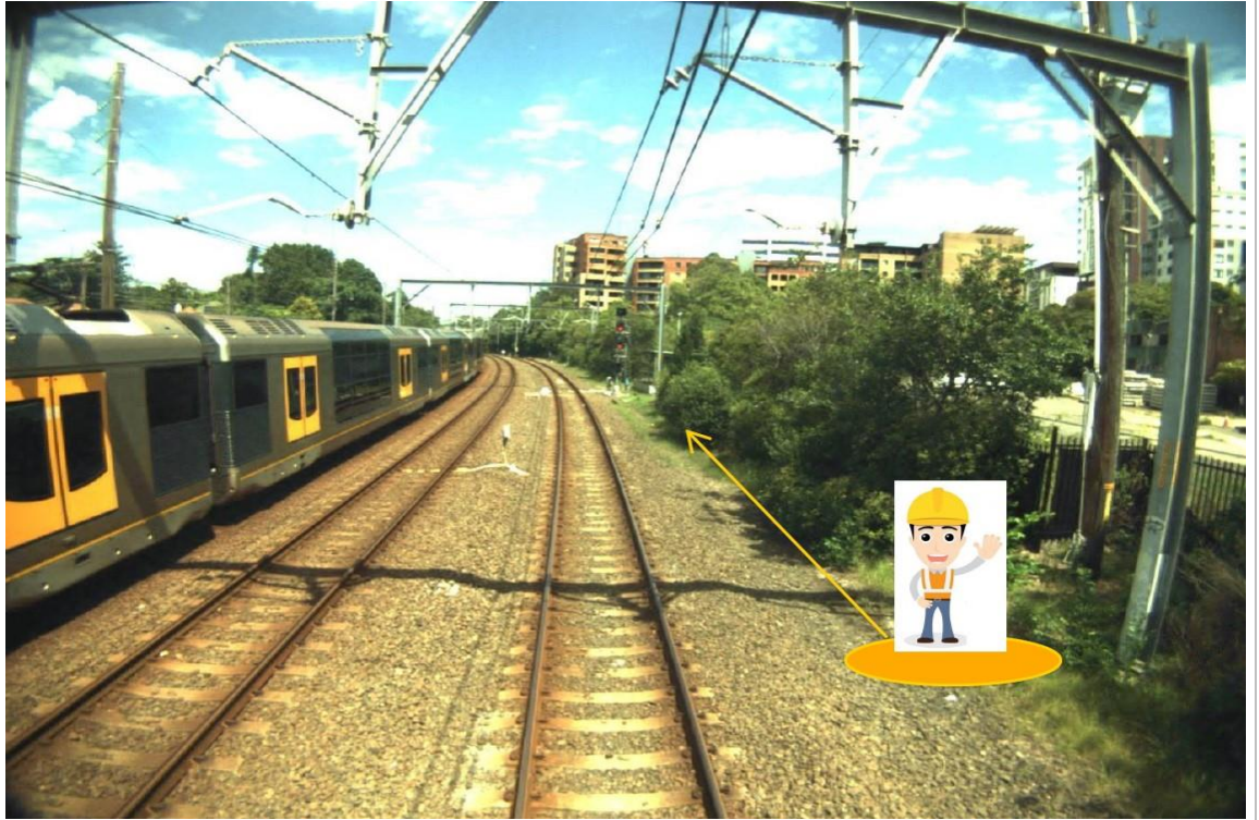
Image 3: Lookout Positioned in designated location at SW15+415 adjacent to Up Illawarra Local , monitoring trains approaching from Penshurst
