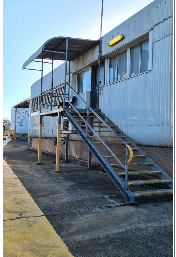
Image 4: XPT Shunters Room
