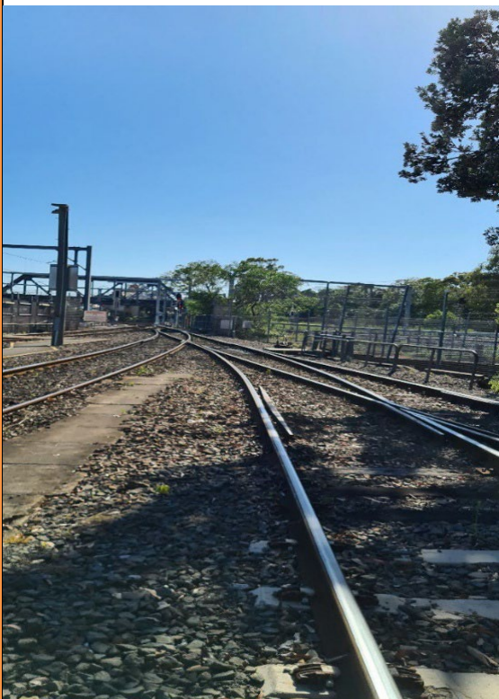
Image 5: View towards City End of XPT Yard
