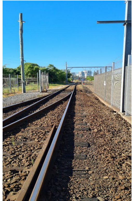
Image 6: View towards Country End of XPT Yard termination Line
