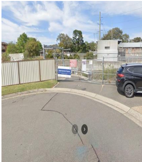
Image 6: Access Gate I20 34.097 D on the Down Side off Caronia Ave
