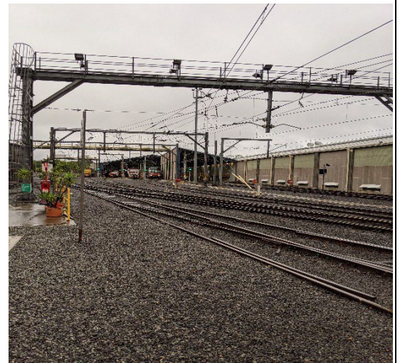
Image 4: Worksite view from the Shunter's office.
