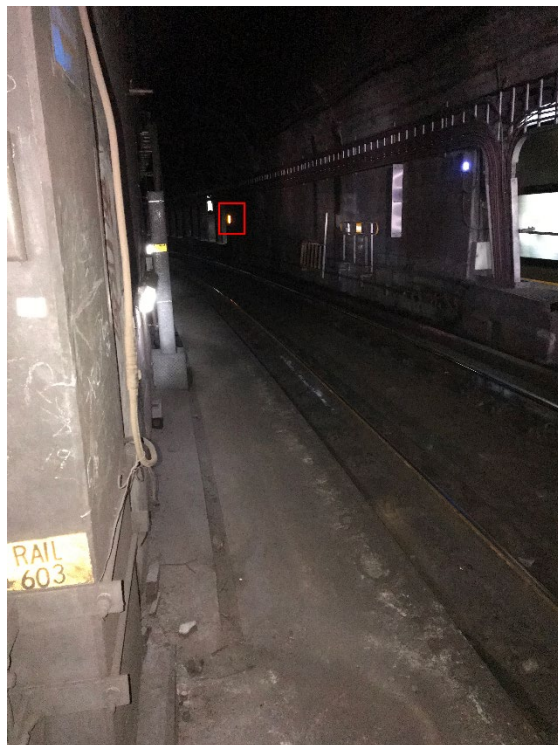
Image 1: Example of warning light at Goulburn Street Portal
