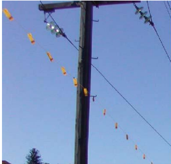
Figure 3: Illustration of a visual tape bunting fitted under overhead power lines
