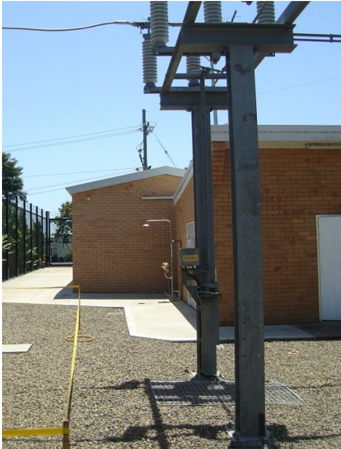
Figure 5: Tape is supported by stands, NOT high voltage structures
