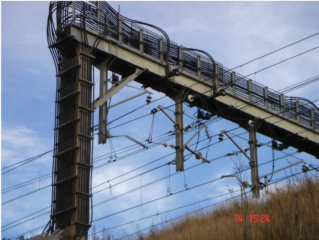
**Figure 3: An example of a feeding arrangement from the Substation to the Overhead Wiring**
