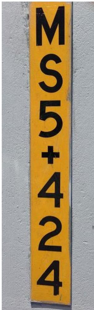
**Figure 6: Example of an OHW structure number label**
