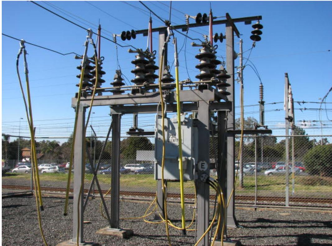
Figure 1: Example of Installed Substation Earthing Set
