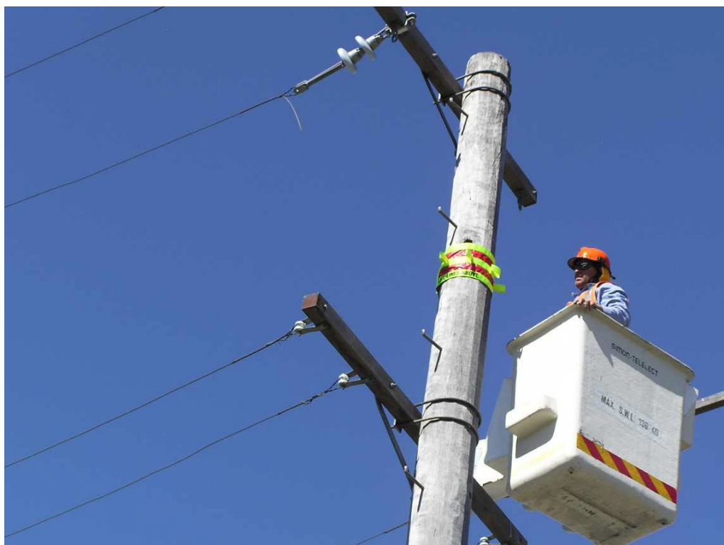
Figure 3: Applying the pole marker from EWP
