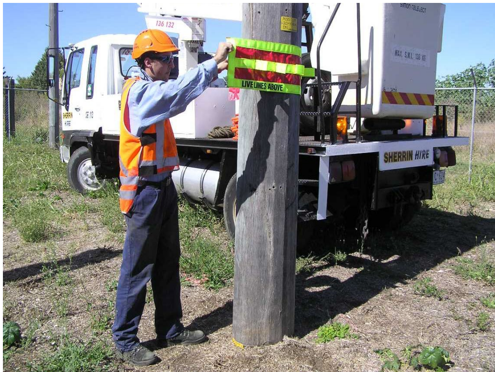
Figure 2: Applying a pole marker at normal eye-viewing height
