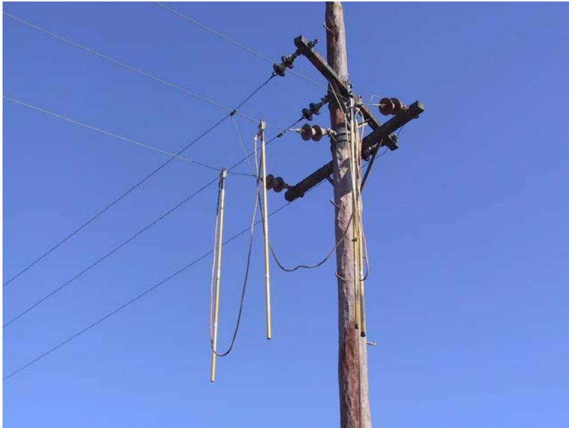
**Figure 5: Earthed aerial conductors**
