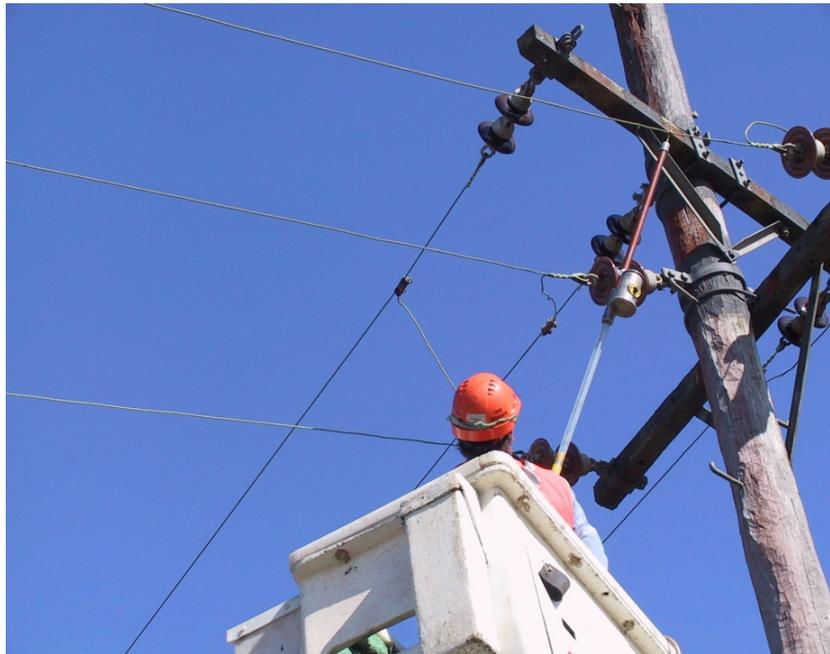
**Figure 2: Testing with High Voltage detector**
