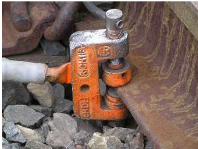
Figure 3: Partially engaged clamp (no good)
