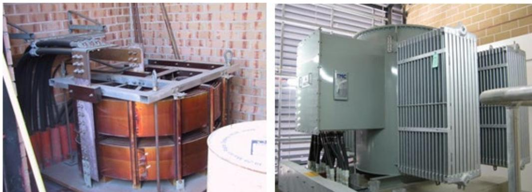
Figure 4: Examples of air and enclosed negative reactors
