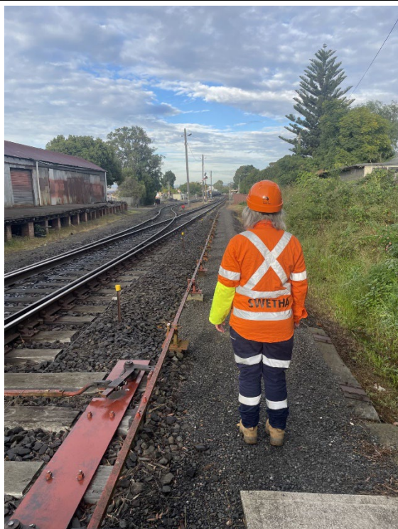
Image 1: View towards End of Terminal Line – Berry end of Worksite (D Frame)
