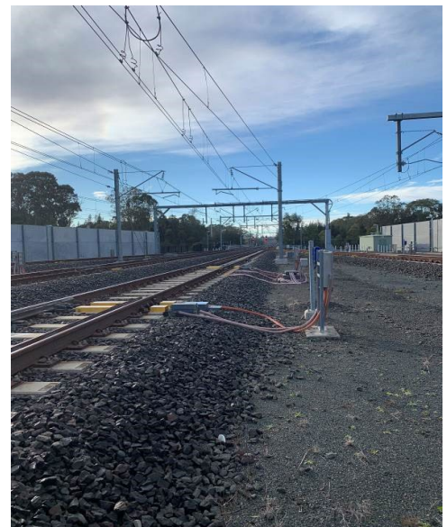
Image 4: View from Leppington yard towards Leppington station.
