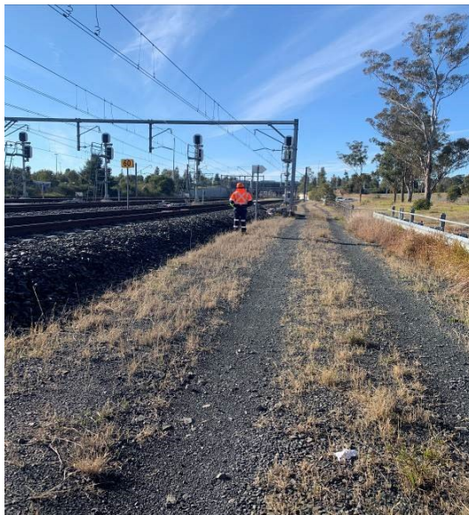
Image 1: Down cess near LE 31 signal towards Leppington Station.
