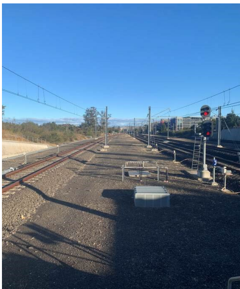
Image 3: View from countryside of Leppington station towards Leppington yard.
