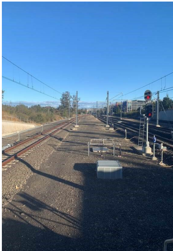
Image 5: view from countryside of Leppington station towards Leppington yard
