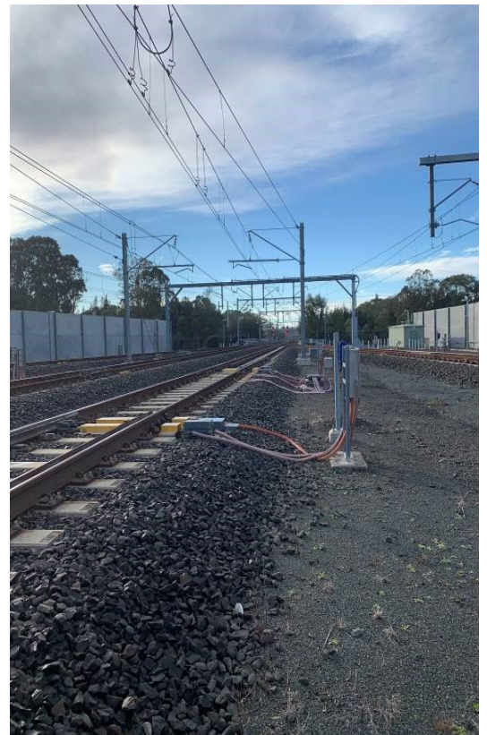
Image 6: View from Leppington yard towards Leppington station
