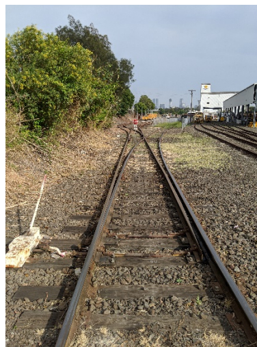
FIGURE 1: Points clipped and locked to prevent rail traffic entry onto the siding
