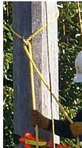
Figure 6 – Rescue rope over pole step, around pole with the tail looped over first pole step
