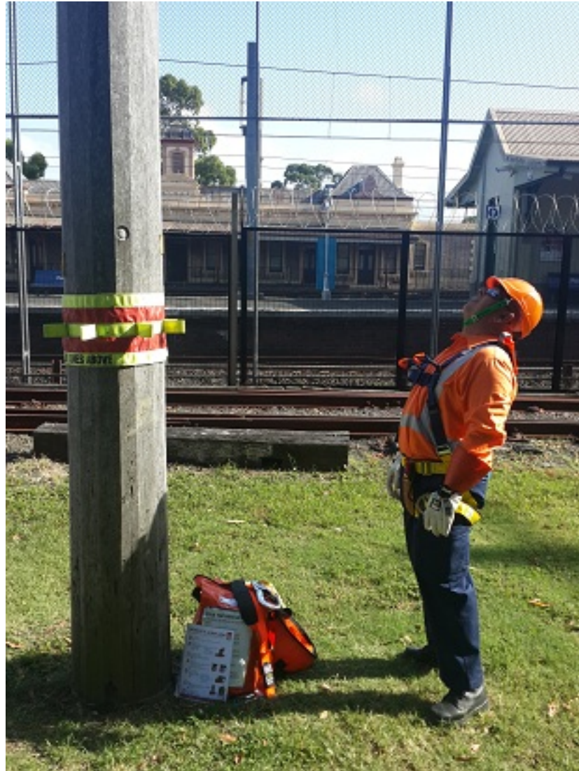
Figure 3 – Accompanying Person Observing with Pole Top Rescue Kit Ready for Use
