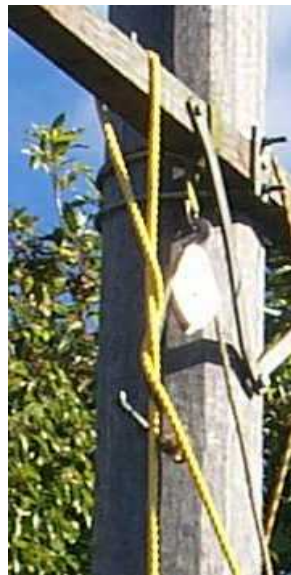
Figure 5 – Rescue rope over cross arm with tail one turn around fall of rope
