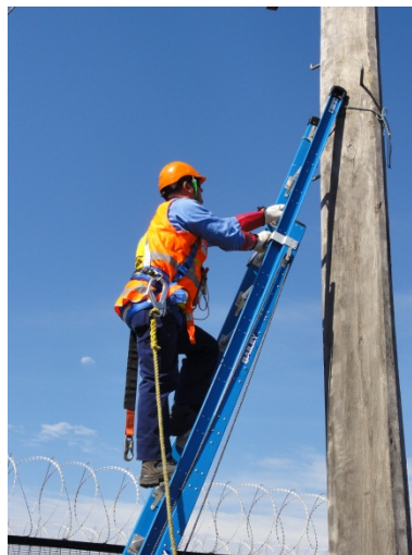
Figure 4 – Accompanying Person Ascending Pole for Rescue
