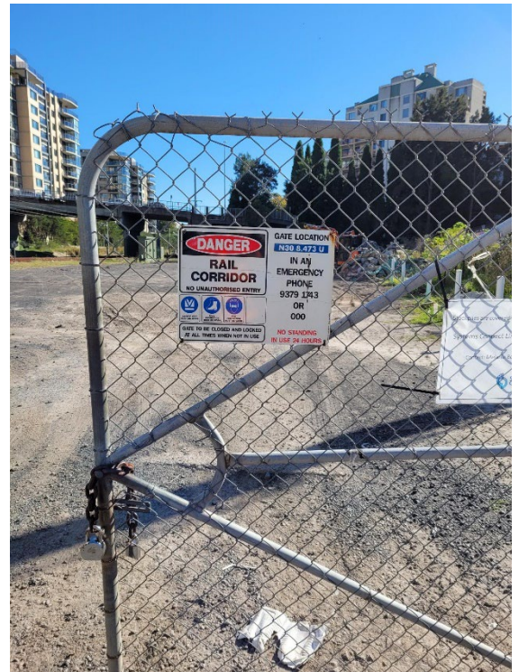
Image 2: Access gate N30 8.473 U
