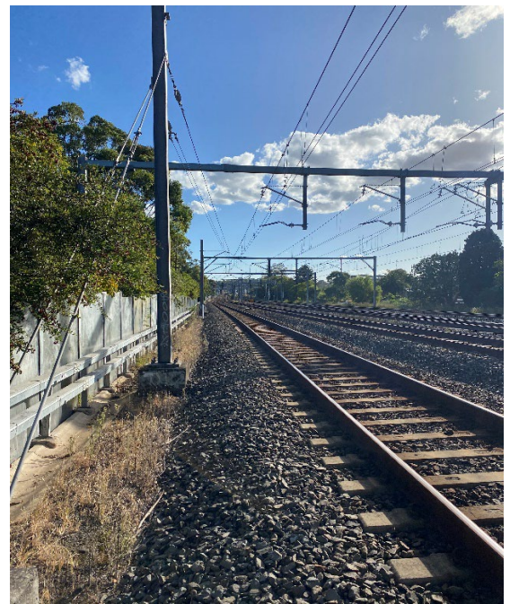
Image 2: View of worksite towards Revesby station
