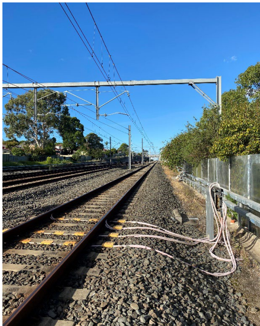
Image 1 View of worksite towards Padstow station
