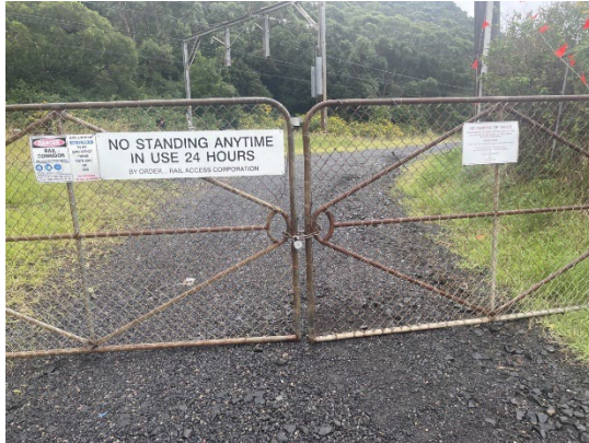
Image 1. Worksite Access City Side of Coalcliff Station (Lawrence Hargrave Dr)
