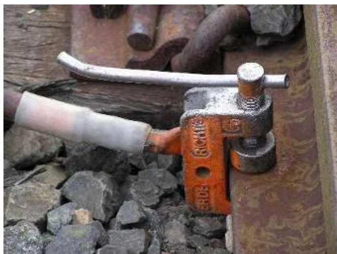
Fully Engaged Clamp
