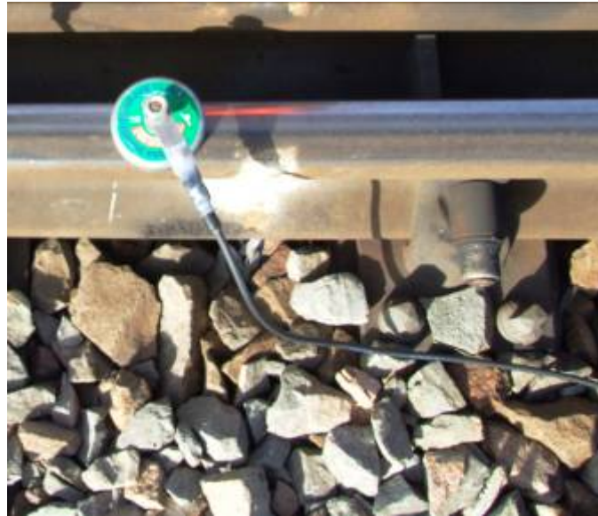
Negative Lug Attached to Welder's Magnetic Clamp
